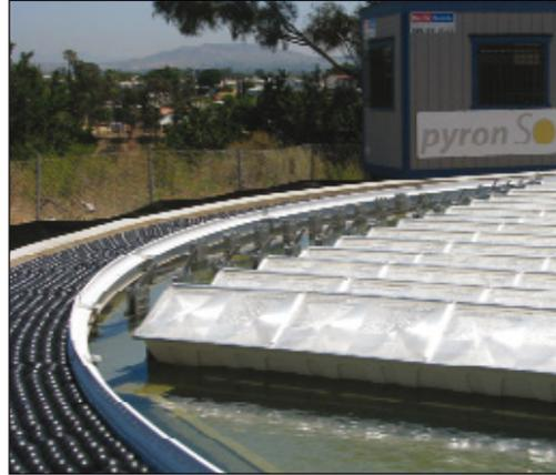
Even more remarkable is the output-to-land ratio, or so-called “footprint” of this new technology. Pyron Solar provides the smallest footprint in the industry, meaning that it requires the smallest area of land per installed MW<sub>peak</sub>; only 3.1 acres are needed to install one MW.
